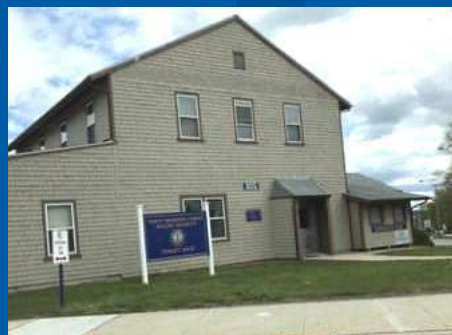
Navy-Marine Thrift Shop. Building 305 on the corner of Peary St and Meyerkord Ave, on Naval Station Newport
